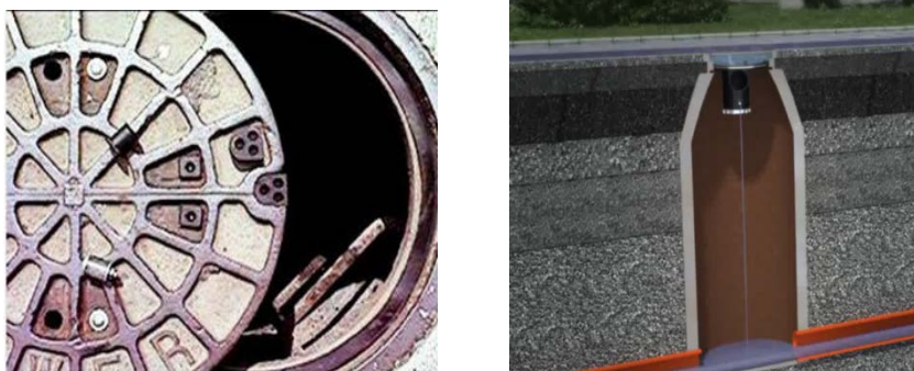
Picture 5 - Some other proposals: using blinding vents in manhole covers, the use of inserts into manholes
